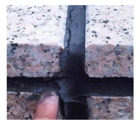
Most of currently commercial PU sealants based on polyether/polyester polyols show limited resistance against ageing
